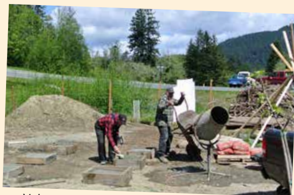
Volunteers pouring foundation for Apple Shack
